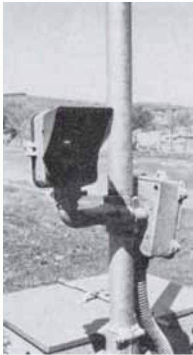
Santa Fe's motor section car indicators operate on the fail-safe system. This particular example in non-CTC territory near Victorville, Calif., shows a small lighted white aspect when everything is clear. Its restrictive aspect occurs then the light goes out, indicating that a train is occupying the block ahead.
