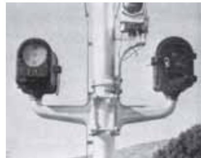
Closeup of Union Pacific indicators near Echo. They indicate train occupancy by having the vertical red dots turn to a horizontal position, obscuring the two green dots at sides.
